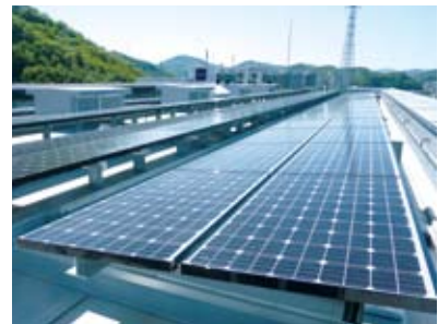
Solar panels installed on the roof of the headquarters building
