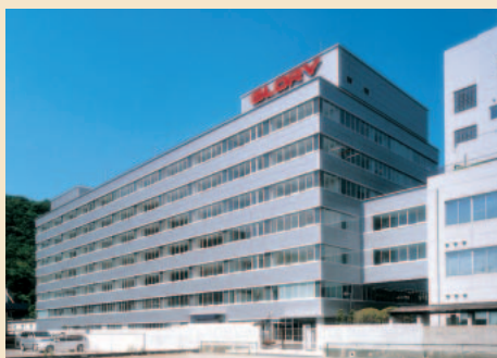
A whole view of the new building---iron-framed, seven stories ---lot area 2683 m 2 ---total floor area 16499 m 2
